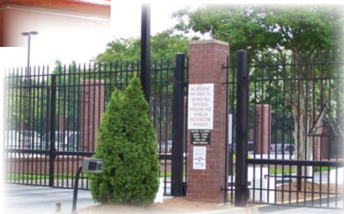
Below: Georgia Power Company's corporate headquarters employee parking deck requires authorized smart cards for entry. Each gate is equipped with the card reader, intercom unit and video surveillance.
